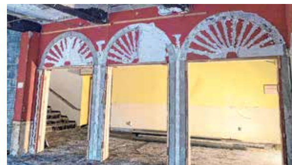
THE ARCHES THAT INSPIRED THE NEW NAME, SUNSET THEATER.
