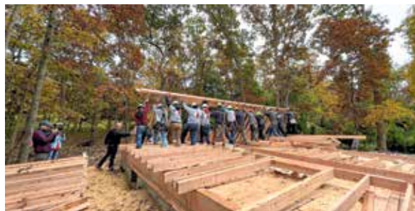
THE REAR WALL OF THE HOME GOING UP.
