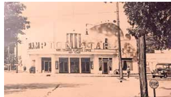
A HISTORIC PHOTO OF THE HAMPTON STAR THEATRE AT SIX CORNERS.
